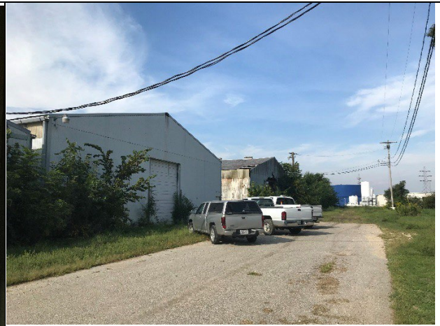
View facing west along W. 9 th Ave. of north end of buildings on Center Parcel.
