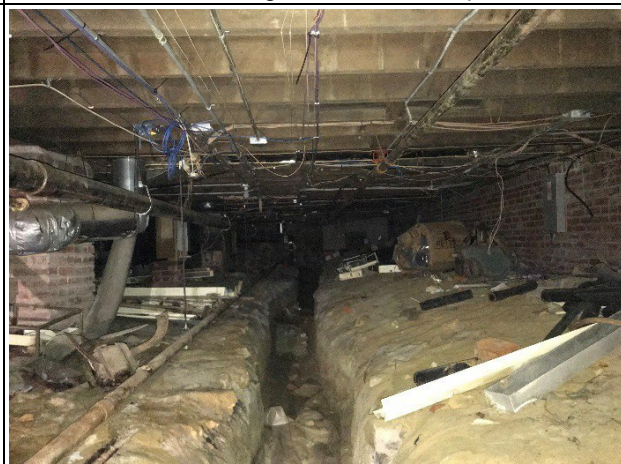
View of crawl space beneath former dry cleaner.
