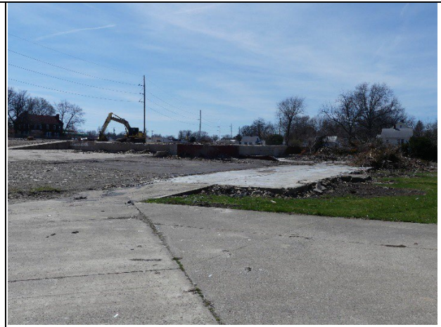
View of site in later phases of demolition.
