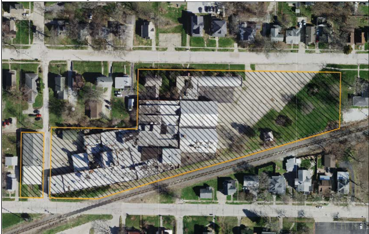
Aerial photograph of site in 2020 prior to demolition of buildings.
