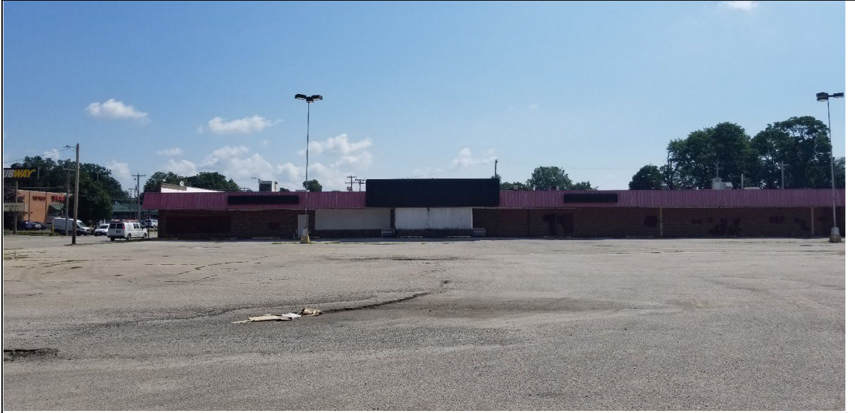
View facing west of former Econofoods store.
