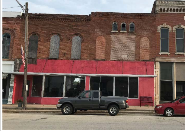
View facing north of the front of the two buildings.
