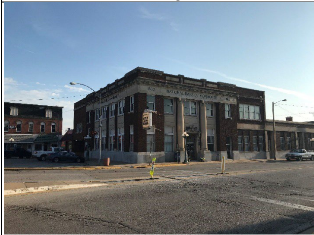
View facing NE of building exterior.
