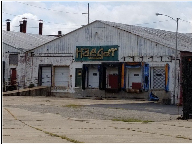
View of buildings (pre-demolition)
